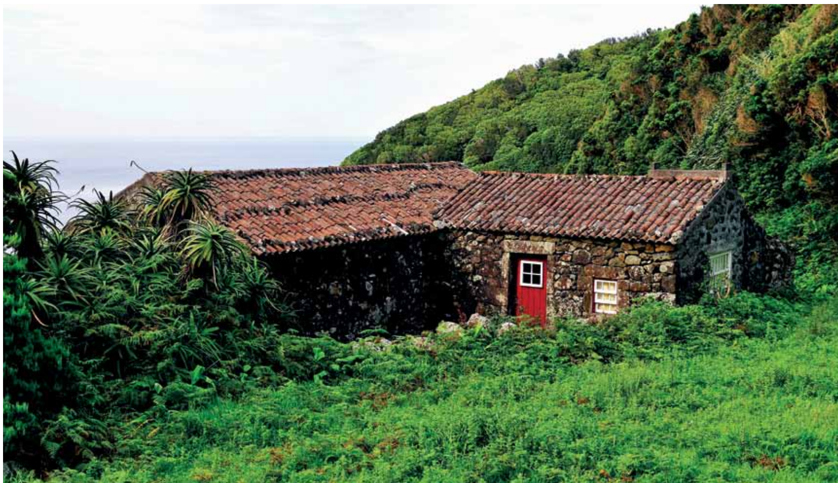
Figure 23. Typical L-shaped house, Fajã da Caldeira de Cima
