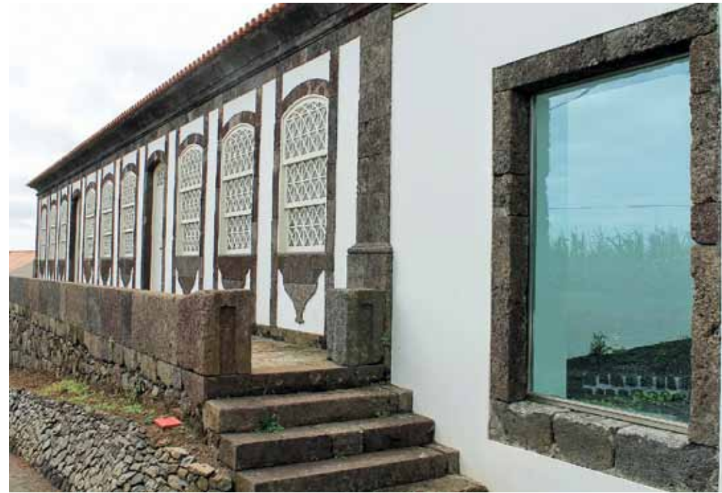
Figure 46. The “Solar dos Tiagos” after restoration, Topo
